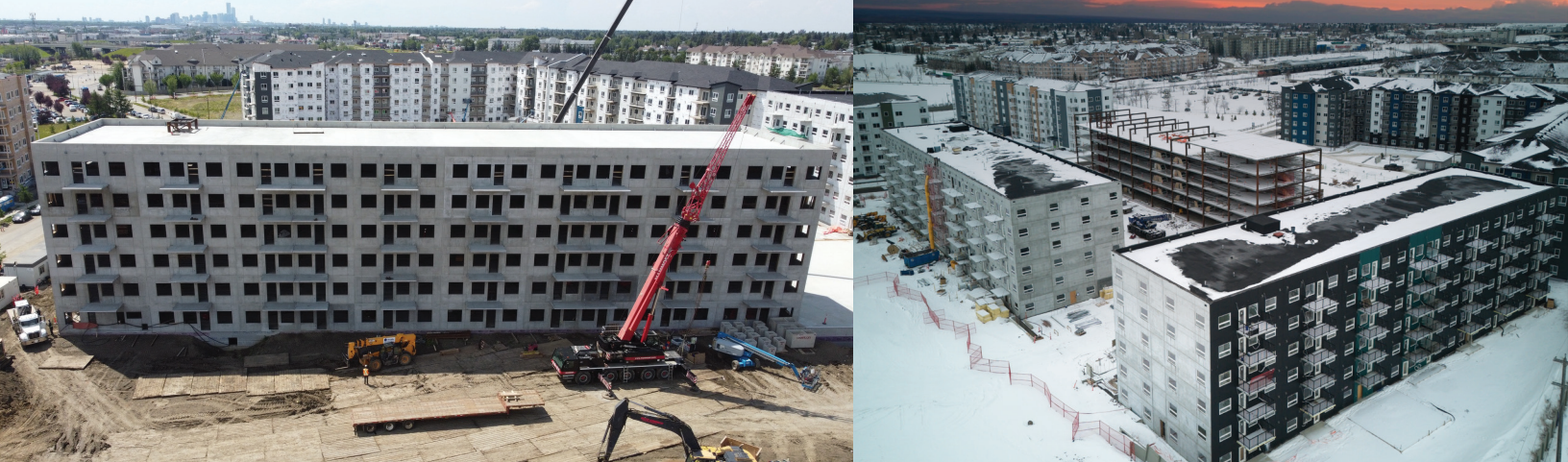
Figure 5-6: Installation of the 6-storey building used in this study.
